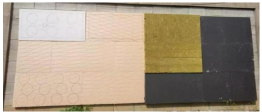
图 4 试验墙铺贴保温板后效果 Fig.4 The effect of the test wall after laying the insulation board
