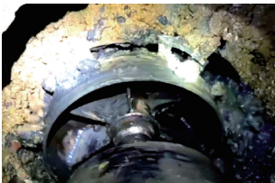
图 7 碎(裂)管设备破碎原有管道 Fig. 7 Crushed (cracked) pipe equipment breaks the original pipeline
