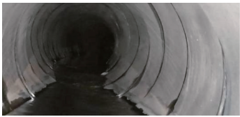
图 8 碎裂管法修复效果 Fig. 8 Repair effect of fragmentation tube method
