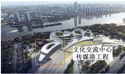
图 1 “一带一路”文化交流中心传媒港公建项目 Fig. 1 “Belt and Road Initiative” cultural exchange center media port public construction project
