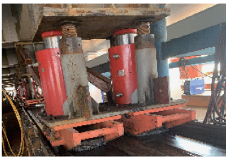
图 6 滑移小车布置 Fig. 6 Layout of slipping cars
