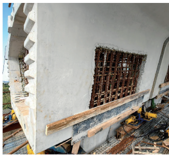
图 15 墩顶块安装 Fig. 15 Installation of pier top block
