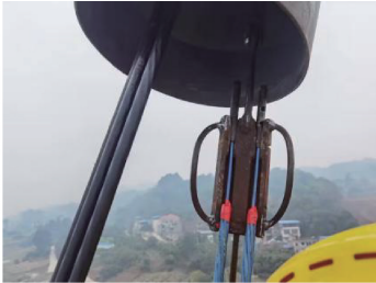
图 1 塔外循环牵引系统单次牵引 2 根钢绞线 Fig. 1 The circulating traction system simultaneously pulling 2 steel strands in a single operation outside the pylon
