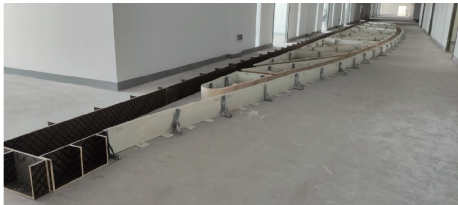
图 3 模板试拼装 Fig. 3 Trial assembly of formwork
