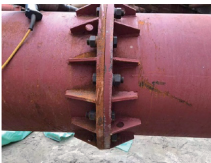
图 6 高强螺栓连接紧固 Fig. 6 Fasten with high-strength bolts
