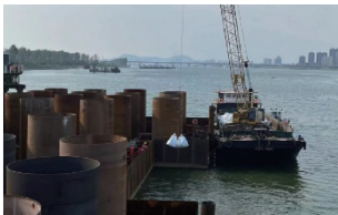
图 12 围堰刃脚封堵施工 Fig. 12 Sealing construction at the cofferdam cutting shoe
