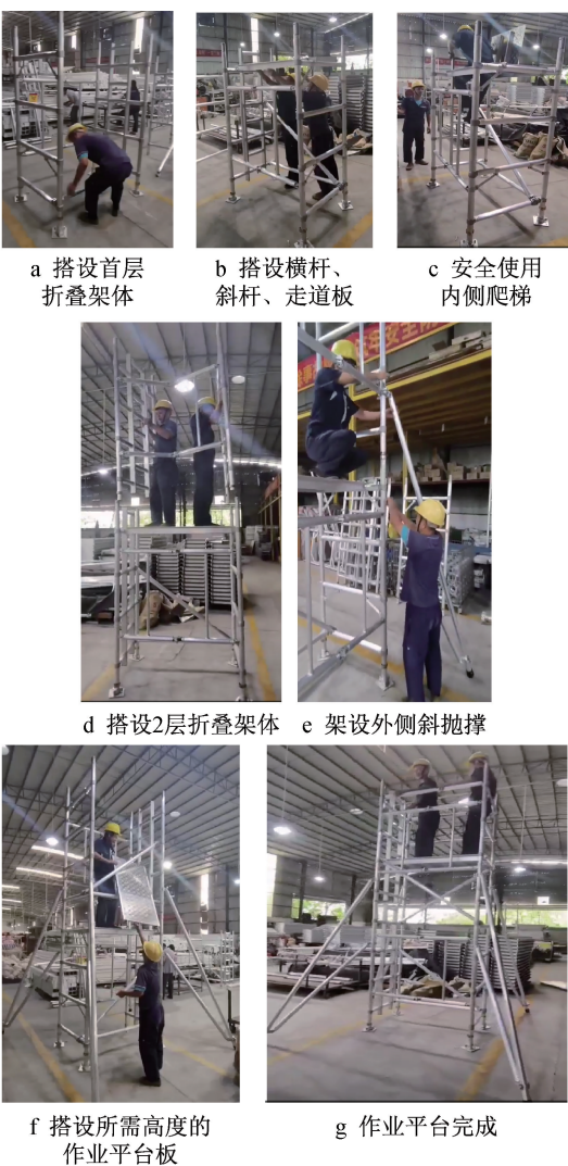
图 6 操作平台搭设过程 Fig. 6 Setting-up process of operating platform
