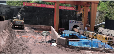
图 3 土斗车编组 Fig.3 Muck car formation
