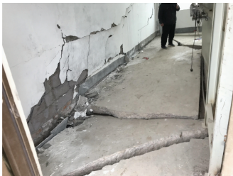
图 13 室内地面沉降开裂 Fig. 13 Settlement and cracking for indoor ground
