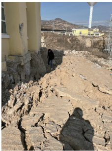
图 7 东侧场地沉降 Fig. 7 Settlement of east side site
