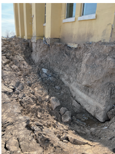
图 9 独立基础外露 Fig. 9 Exposure of isolated foundations
