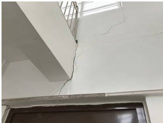
图 12 次梁与框架梁交界处开裂 Fig. 12 Cracking at junction of secondary beam and frame beam
