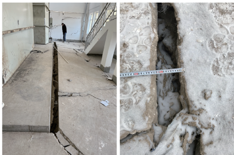
图 10 场地地面及室内地面开裂 Fig. 10 Cracking for site ground and indoor ground
