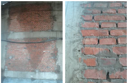
图 3 墙体竖向裂缝 Fig. 3 Vertical cracks in the wall
