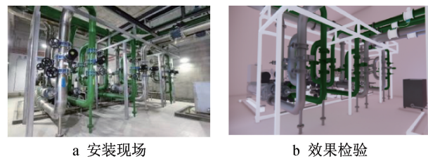
图 13 装配式冷水机房安装现场及 BIM 效果检验 Fig. 13 Installation site and BIM effect test of prefabricated cold water room
