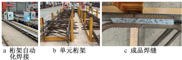
图 11 桁架焊接平台加工、堆放单元桁架 Fig. 11 Truss welding platform processing and stacking unit trusses
