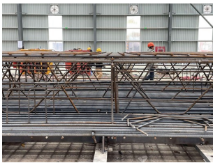
图 12 采用桁架单元制造的钢筋笼 Fig. 12 Reinforcement cage made of truss element
